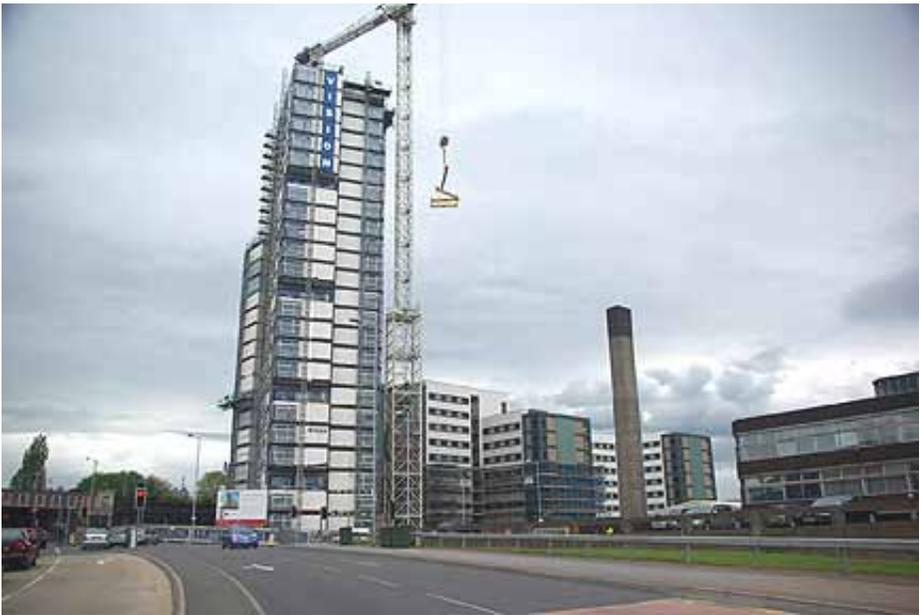
*Pictured left: Europe’s tallest modular building—a \$34 million UK project. Designed by O’Connell East Architects of Manchester, the 24 story student dormitory is made up of 805 modules and designed to be built in 27 weeks.*
