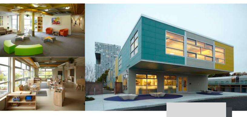
MIT needed additional space for childcare as an addition to the Cambridge campus. The project required a short timeline, and they turned to Triumph Modular as a leader in modular construction to help. The 14,000-square-foot steel and concrete building was fabricated in Pennsylvania and shipped to Cambridge.
