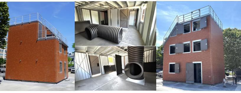
The City of Cambridge Fire Department, in partnership with WHP Manufacturing and Triumph Modular, completed the construction of a custom fire training facility adjacent to Fire Station Engine #3. This three-story, 960-square-foot auxiliary building, fabricated from galvanized steel, was designed for realistic fire simulations, with replaceable components to withstand heavy use. To match the aesthetics of the existing firehouse, the structure was finished with brick veneer siding.
